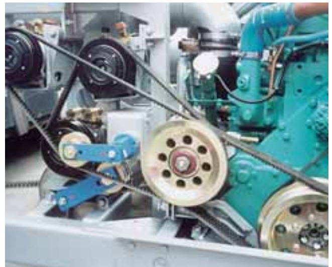
Belt tensioner on belt drive between diesel engine and an alternator
